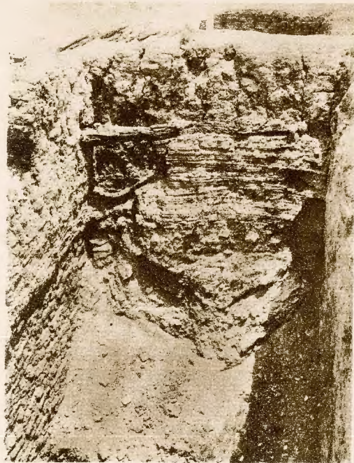
C. EVIDENCE OF MAGAZINE ROOFING.
